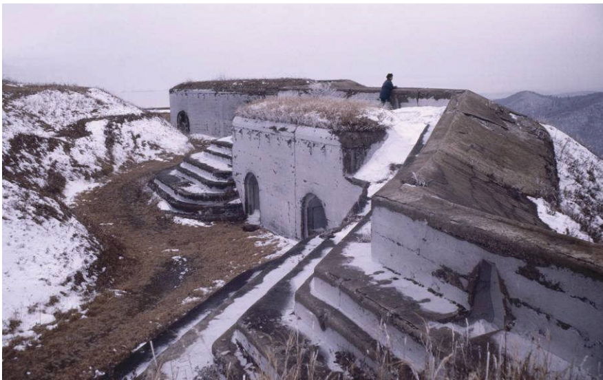
Fig. 5.5. Fort # 4. A rifle parapet and exits from the gallery beneath the parapet
