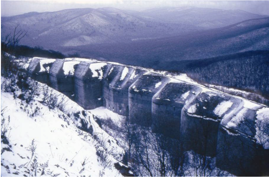
Fig. 5.4. Fort # 4, 1910-1917. Military engineer E. Protsenko. A double counter-scarp caponier (coffre) in the ditch
